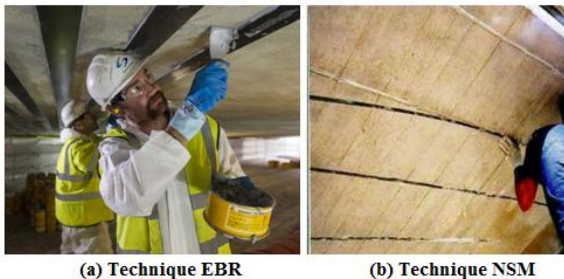
Figure 1. 10. Techniques de renforcement. [20]
