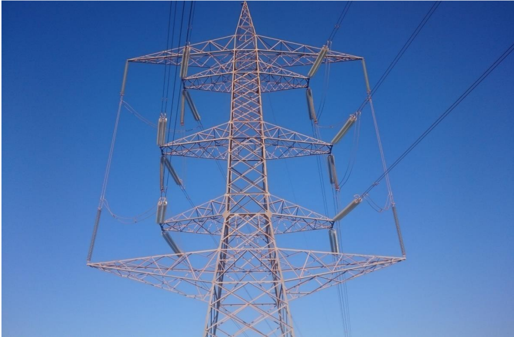
Figure IV.8 Transposition de phases
