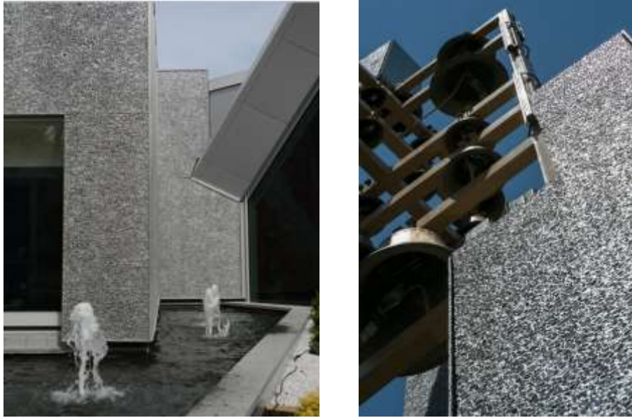
Figure I.21 Aluminum foam used for construction projects (ALUSION by Cymat Technologies Ltd).
