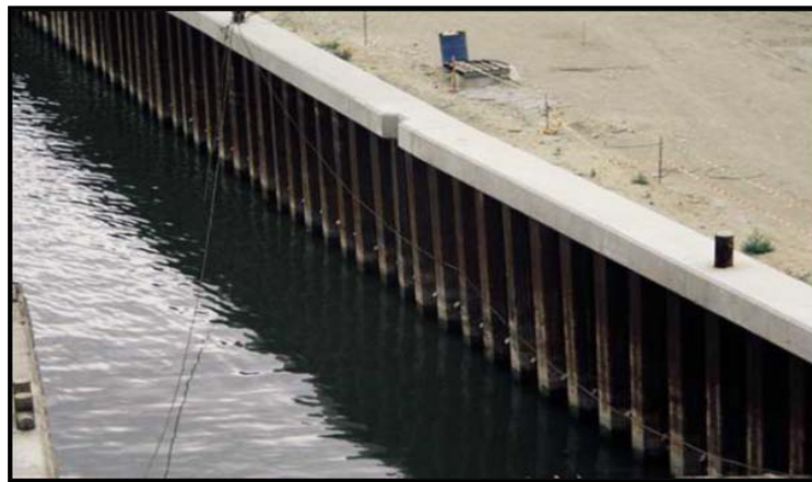
Figure I.10 Les rideaux de palplanches. [30]
