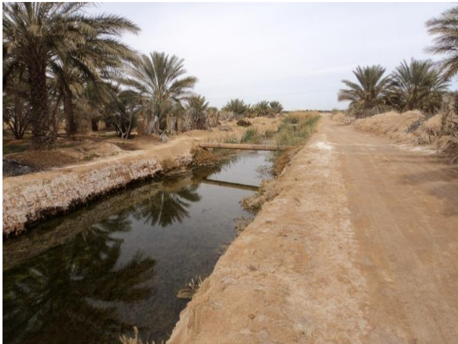
Figure 4 : Drains de Zaouia Labedia (2011, Touggourt)
