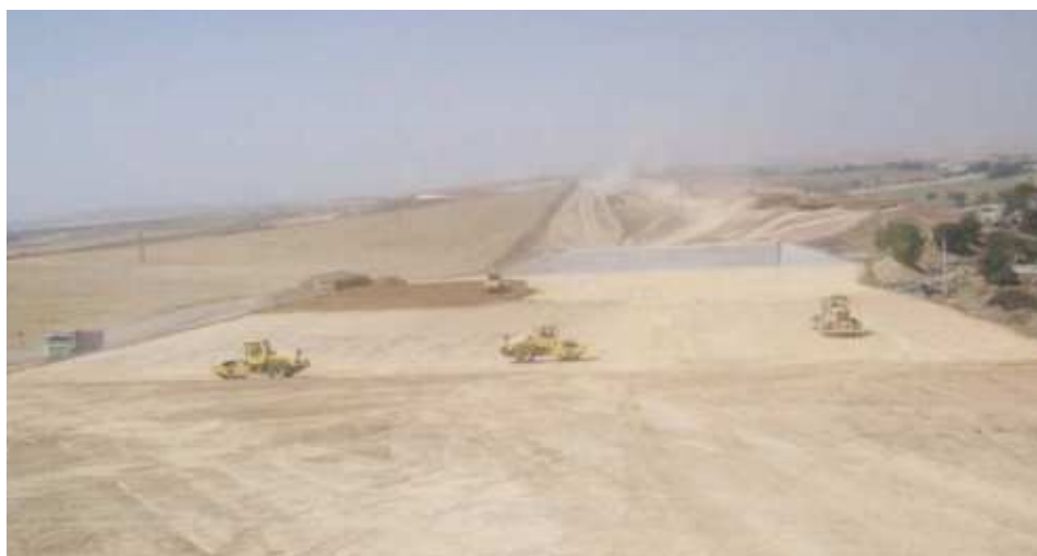
Photo A.4 : section remblai constantine, comp3
